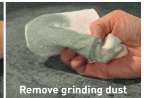
Remove grinding dust
